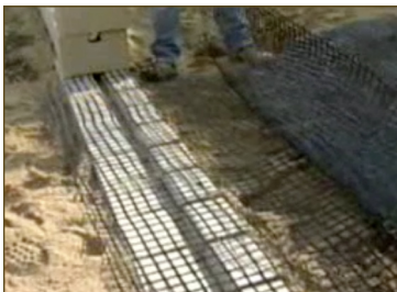
Diagram 9—Geosynthetic Reinforcement
